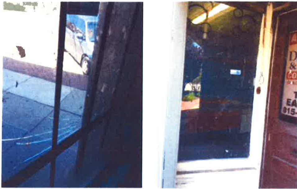
Replacement of busted plate window next to downstairs entrance.
