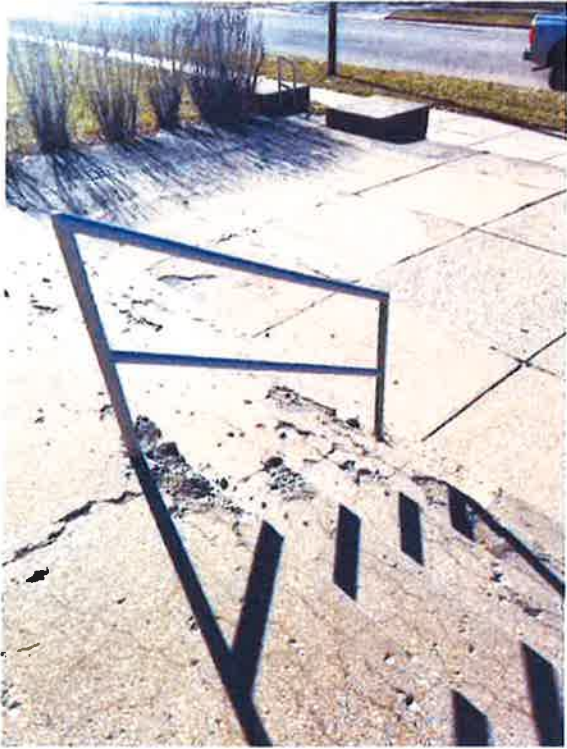
Photos of area to be repaired
