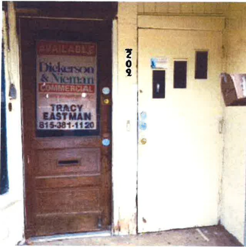
Replace two front doors
