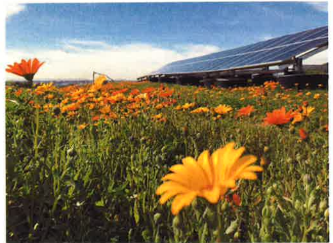
Vision: Ballasted Solar Project
