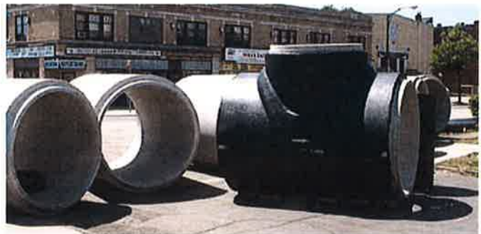
Installing storm sewers. Source: http://www.erdmananthony.com/ProjectPortfolio/Detail.aspx?id=41
