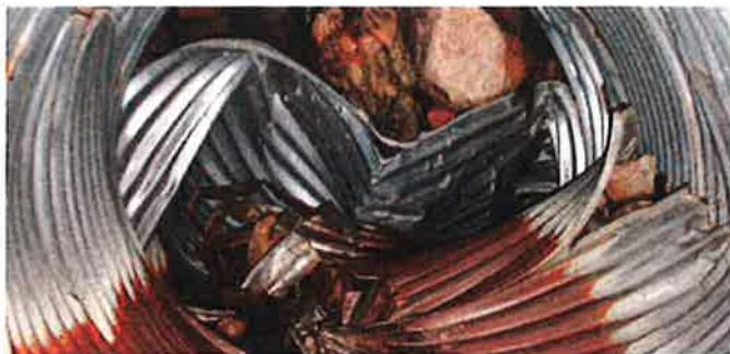
Replacing failing culverts. Source: www.newnhamfarms.com
