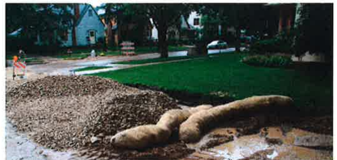
Upgrading local drainage. Source: http://saveourstream.blogspot.com/p/green-infrastructure.html
