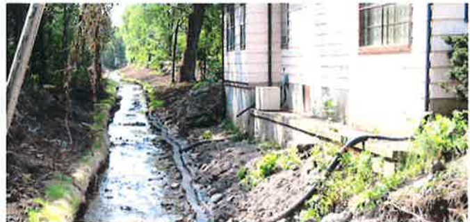
Stabilizing streams and other stream restoration projects.
