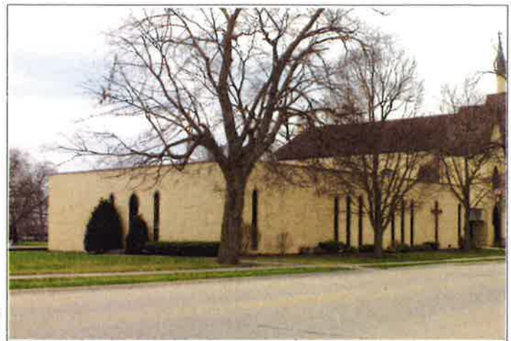
Photo: 221_N_Main_St_SURVEY_Photo_Fellowship_Hall.tif Description
