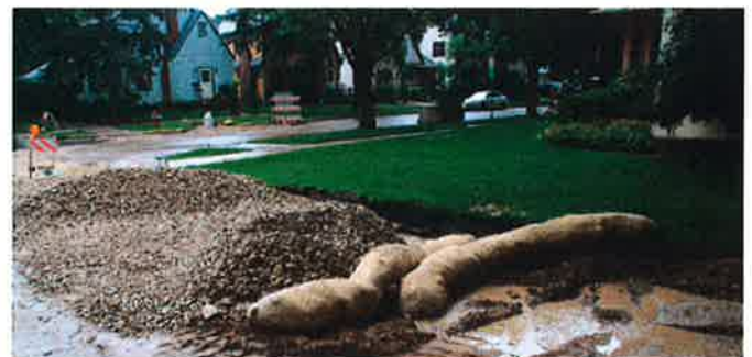
Upgrading local drainage. Source: http://saveourstream.blogspot.com/p/green-infrastructure.html
