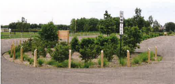
Implementing green infrastructure projects.
