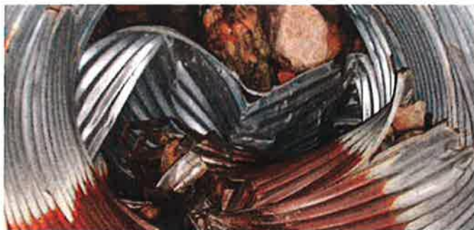
Replacing failing culverts. Source: www.newnhamfarms.com
