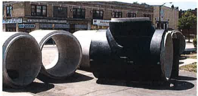
Installing storm sewers. Source: http://www.erdmananthony.com/ProjectPortfolio/Detail.aspx?id=41
