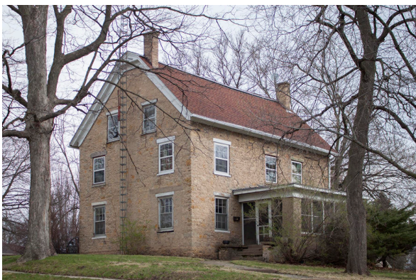
Figure AS1. Stone House. 424 N. Main Street
