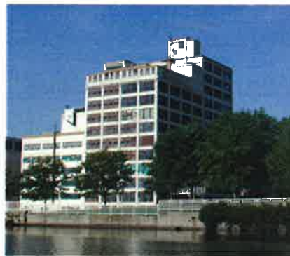
Ziock Building, 1912, Rockford
