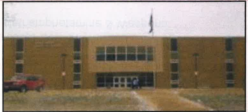
Belvidere High School, photo courtesy of district100.com
