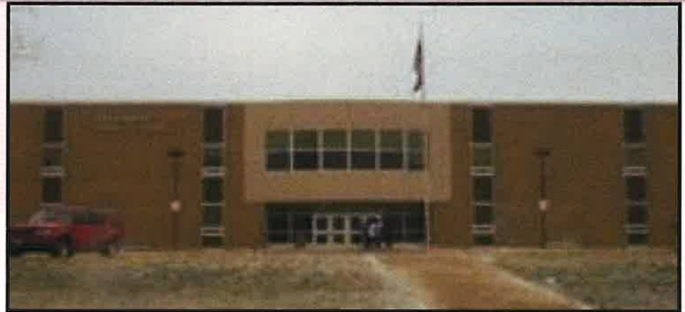
Belvidere High School, photo courtesy of district100.com
